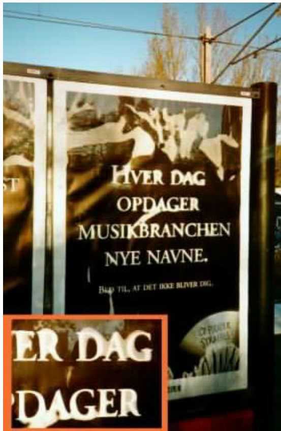
Figure 2. The condensation behind the glass covering a poster is concentrated over the white parts of the image.
