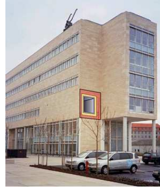
Figure 20: A building of Copenhagen University, holding the archive of the Arnamagnæan Institute. The end wall of the archive is removed to show schematically the heavier insulation towards the interior of the building, the massive concrete wall and the cellular concrete humidity buffer.
