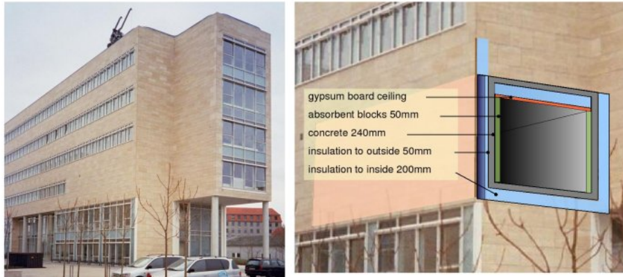
Figure 8: The Arnamagnaean archive of Copenhagen University lies behind the windowless section of the facade. The close up on the right shows a section through the archive. Notice the unusual placing of insulation against the interior of the building and the thinner insulation on the external wall. Humidity buffering of the empty room is provided by 50 mm of cellular concrete lining the interior. It is finished with porous silicate paint to prevent dusting.
